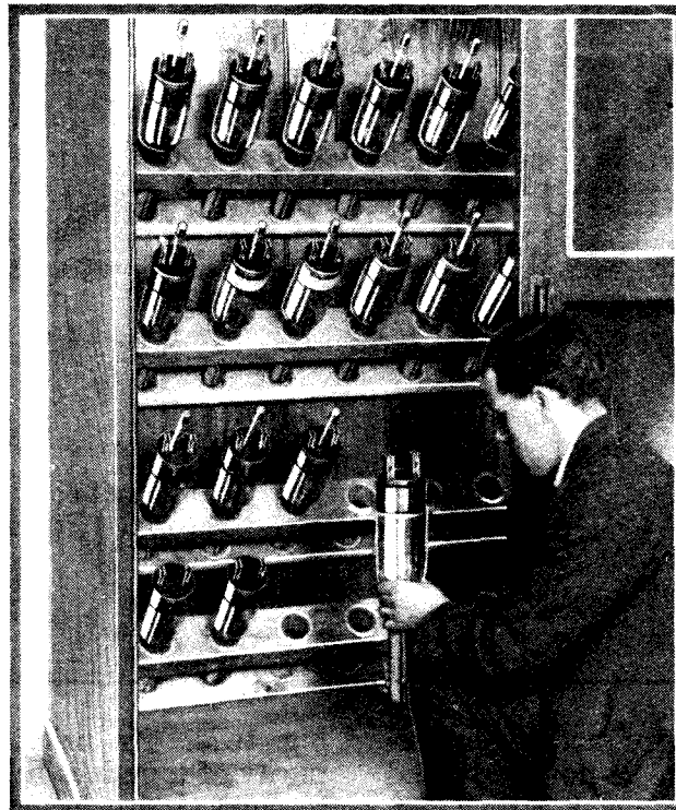
How valves are stored at the Rugby station.
